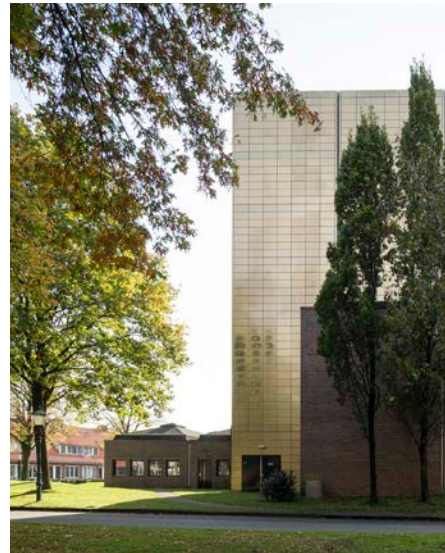
Rear side of the Flint along Plantsoen
